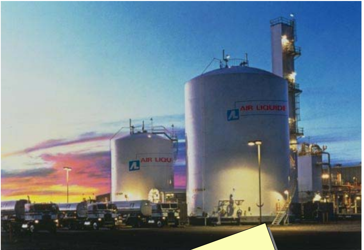
Photo: Air Liquide
