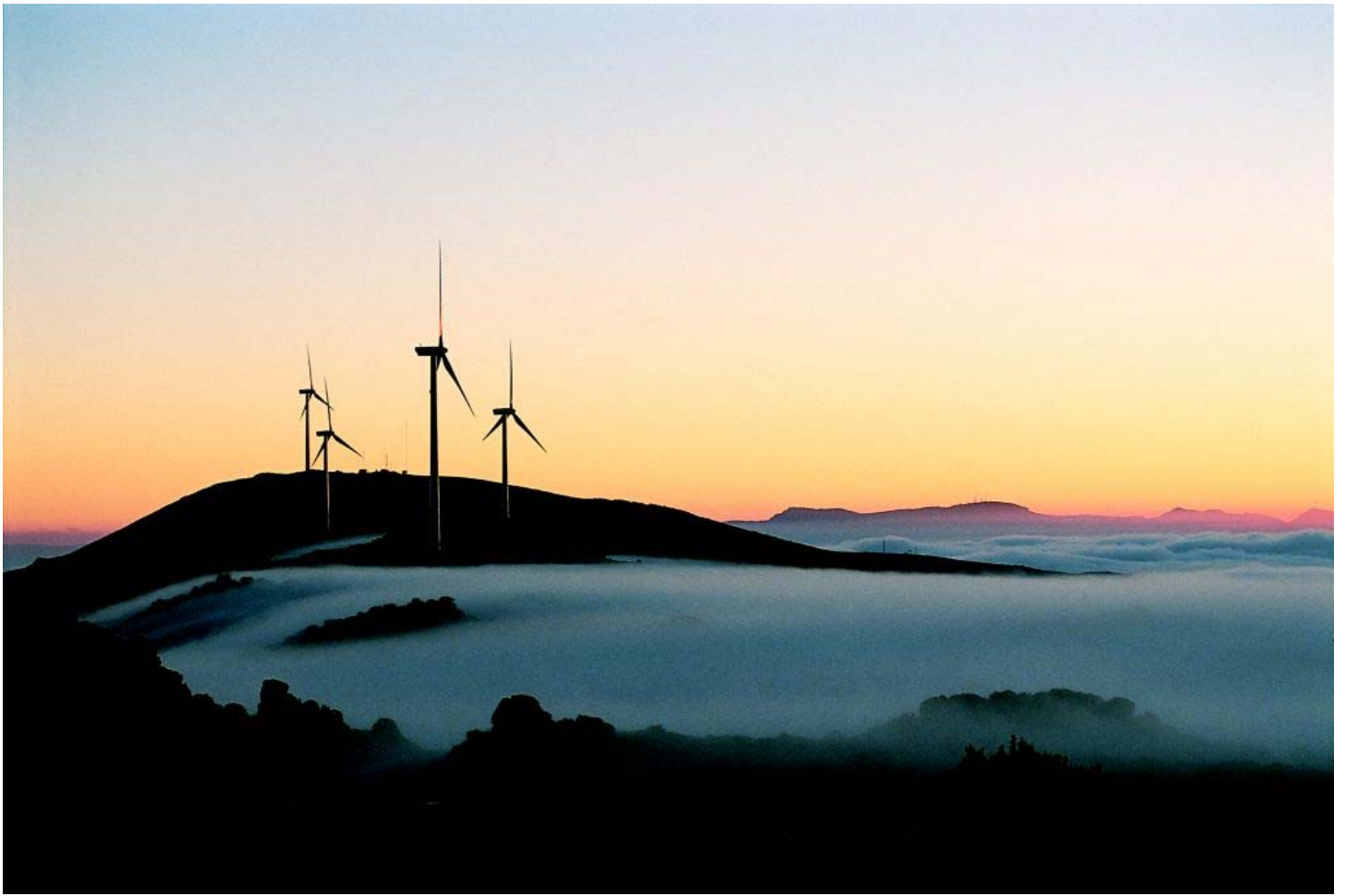
V80-2.0MW & V90-3.0MW Meroicinha Portugal Courtesy of Vestas Wind Systems A/S
