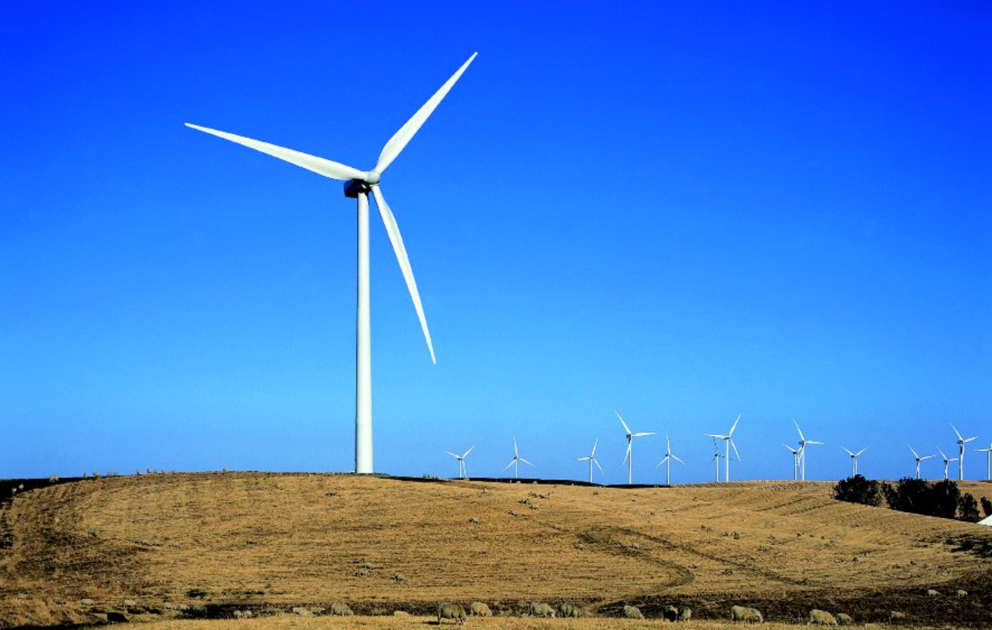
81x V80 – 1.8MW High Winds, California Courtesy of Vestas Wind Systems A/S
